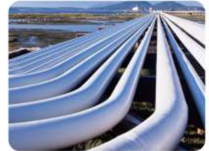
CROSS COUNTRY PIPELINE
